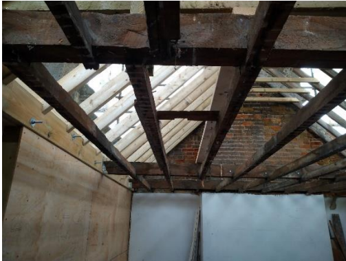
New roof structure, Marine Gardens
