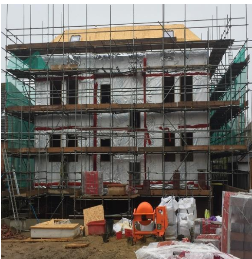
Folkestone – New Build 14 Apartments
